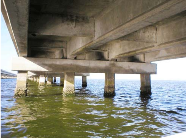
1950's Approach Spans Girder on Pile Cap-Type Pier
