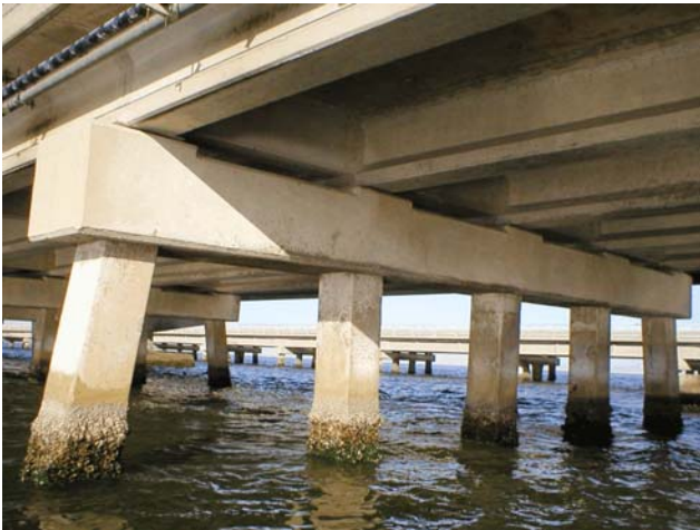
1970's Approach Spans Girder on Pile Cap-Type Pier
